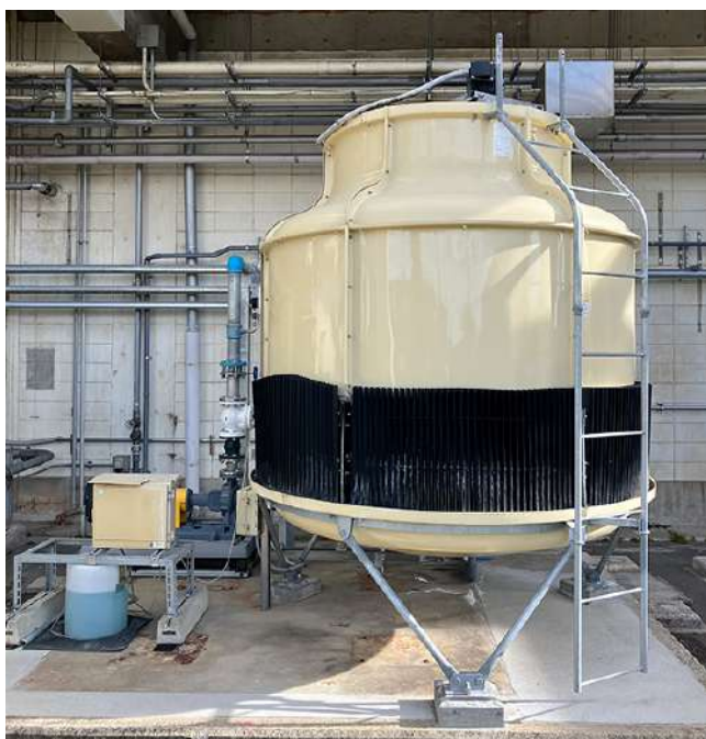
Cooling tower for water-cooled AC at the Chukyo Factory (after consolidation)
